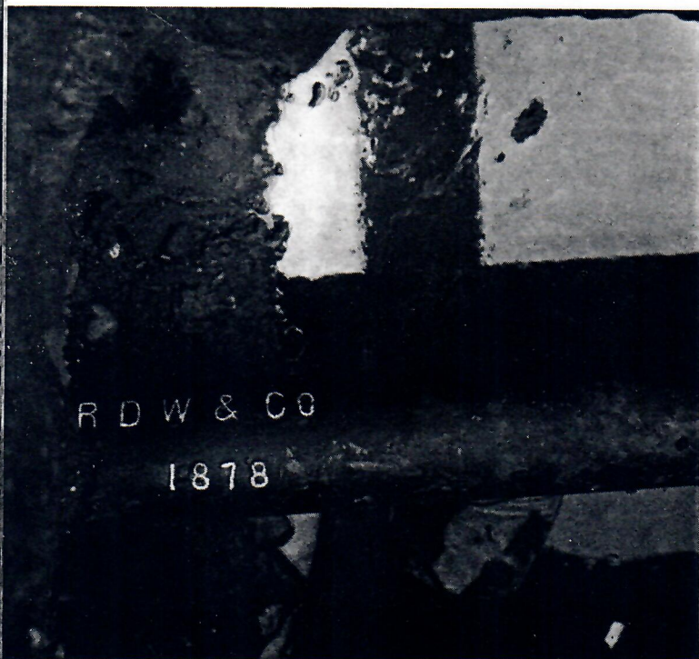
Seventy-five-year-old pipe still in service.
